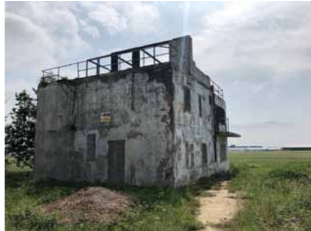
The derelict control tower
