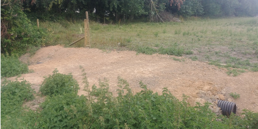
Photograph 5: Recently dug dry ditch and calvert
