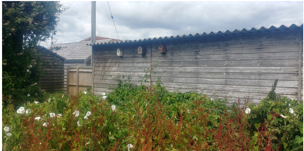
Photograph 2: Three domestic bird boxes located on the rear of building B1
