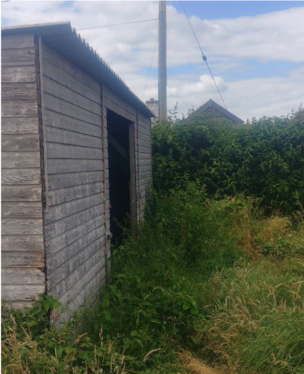
Photograph 1: Building 1 located within the south-west corner of the site.
