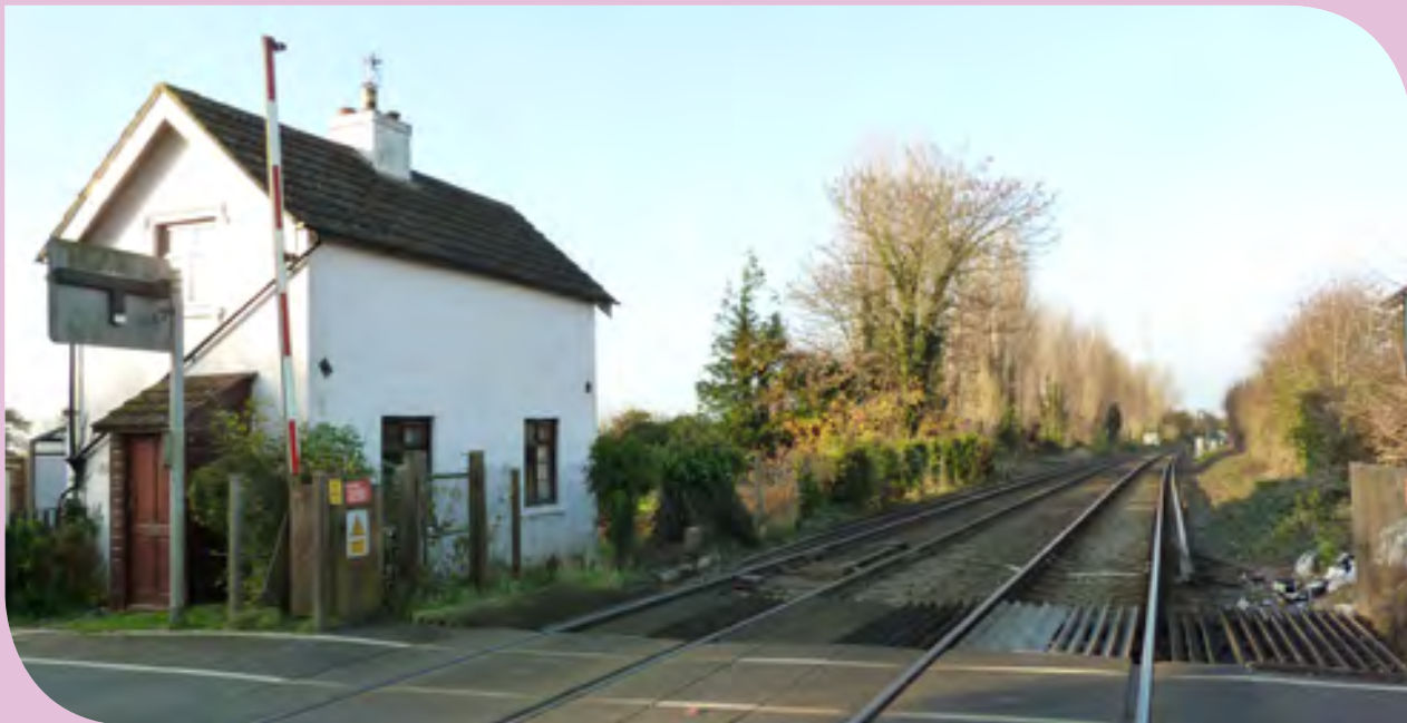
Existing Inlands Road level crossing (site on right)
