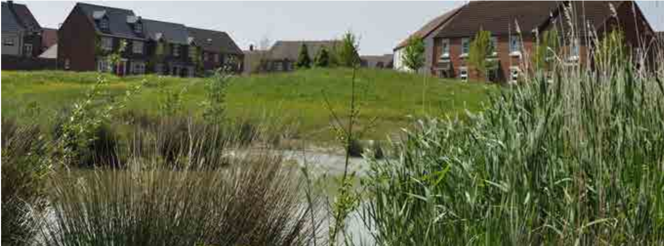
Attenuation features will be provided to create an attractive and sustainable environment
