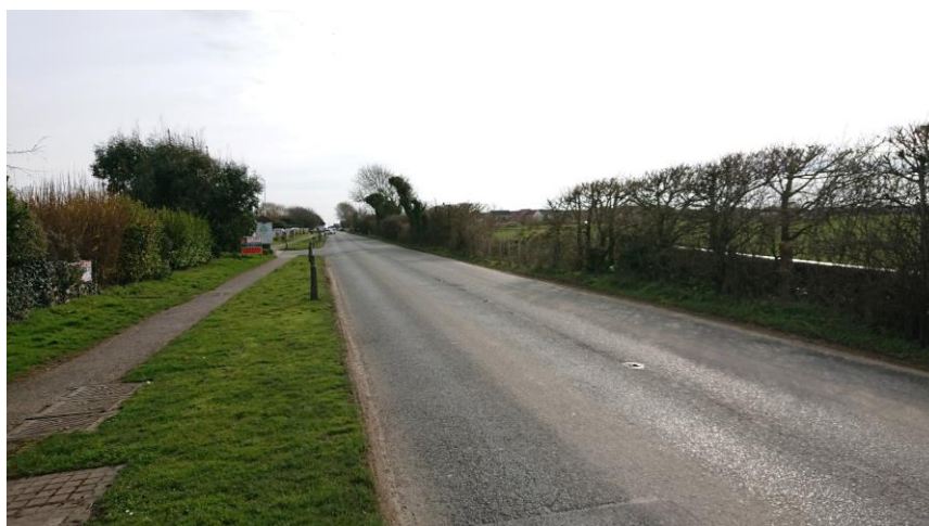
Photograph 1: Conditions on Bracklesham Lane (looking south)
