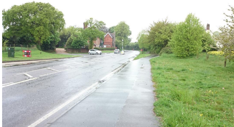
Photograph 3: Pedestrian Conditions on Main Road
