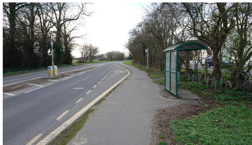
Photograph 4: Bus Stop Conditions
