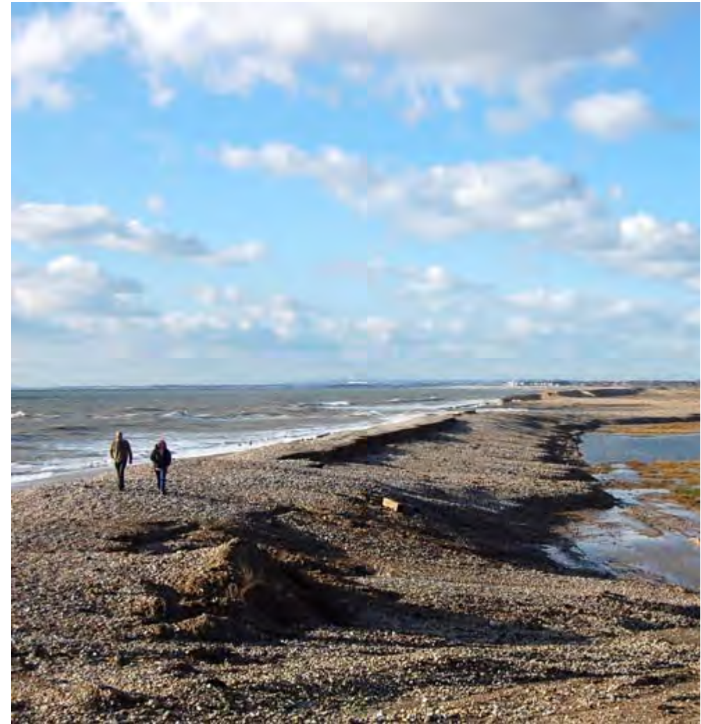
Coastal realignment at Medmerry.
