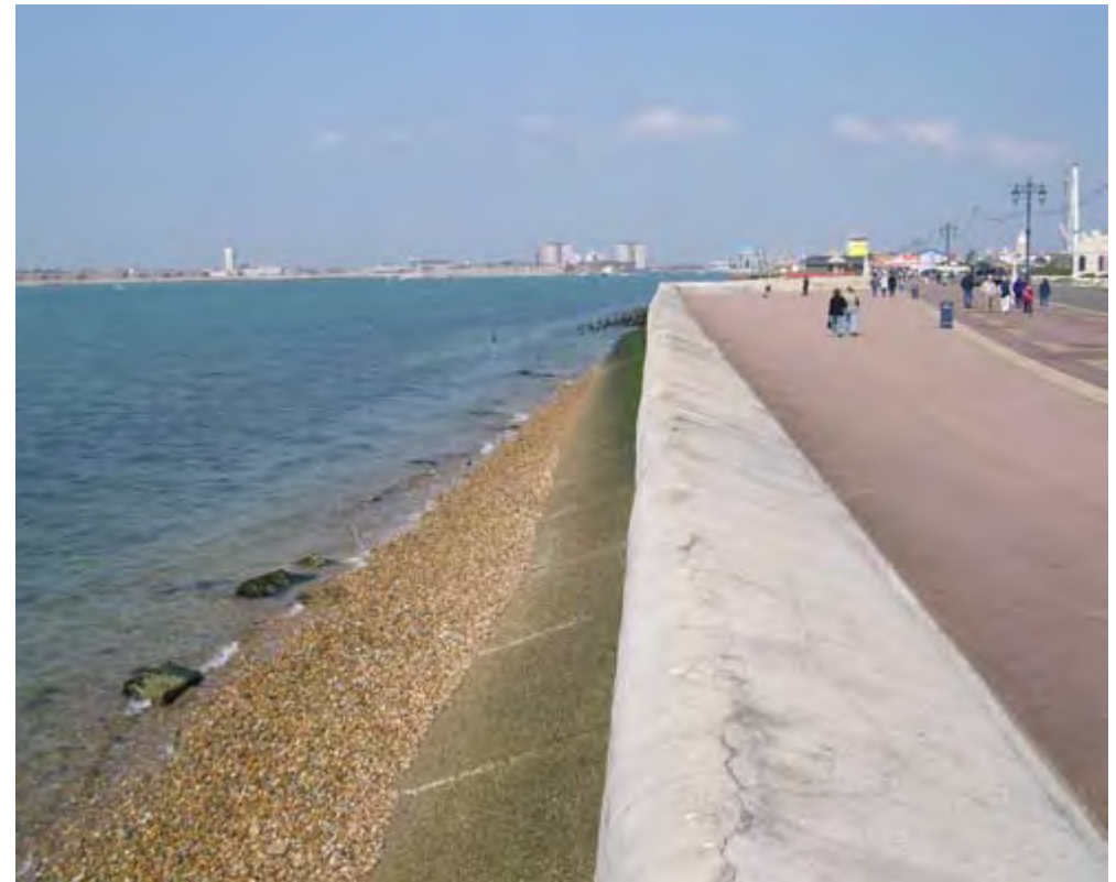
Sea wall at Southsea, Portsmouth.
