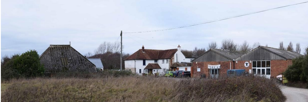
HBA Photo 11 - buildings on the site
