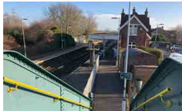
Pedestrian bridge at Bosham Station
