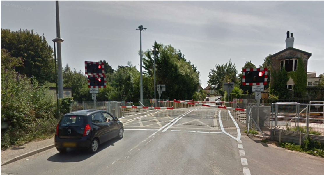
Image 4.2: Yapton level crossing after upgrade
