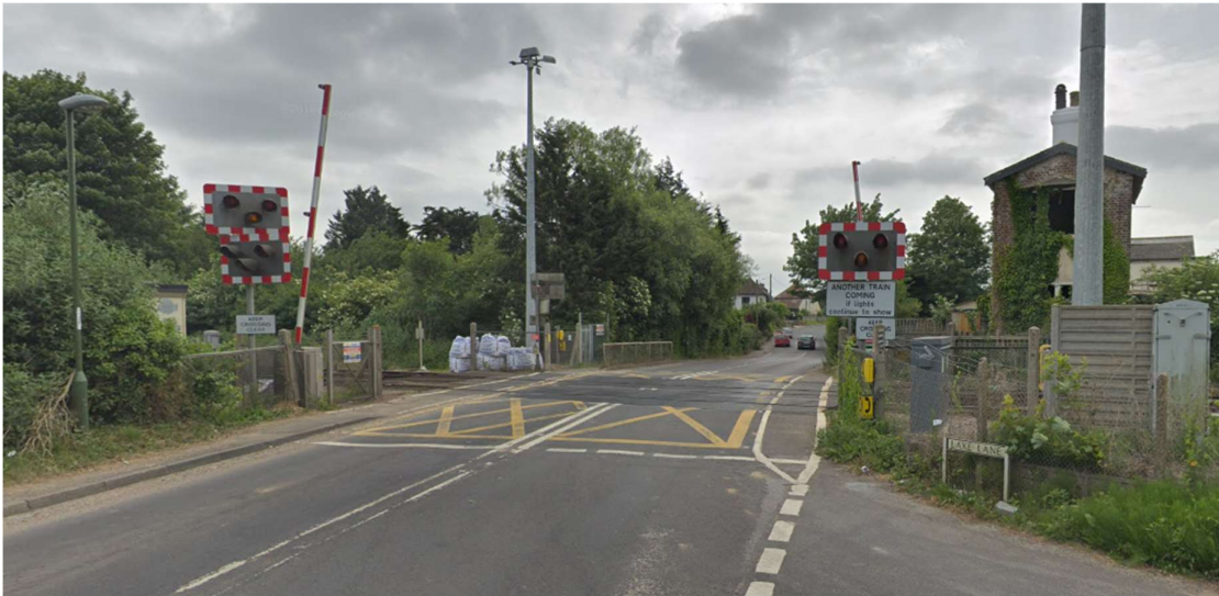
Image 4.1: Yapton level crossing before upgrade
