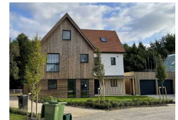
Fig 82: Springfield Meadow is an example of a housing development in Oxfordshire delivered through the use of a panelised MMC system. The MMC system used to deliver the scheme is called the Biond System.
