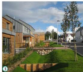
Boardwalks linking over the bioswale alongside the Grove
