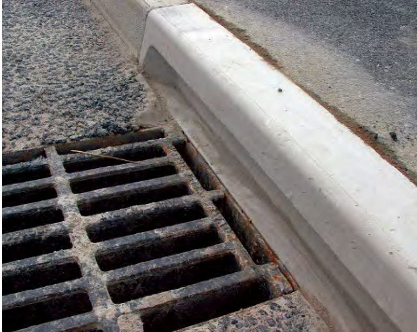
Figure 4: Wildlife kerb to be used on all gully pots within the development
