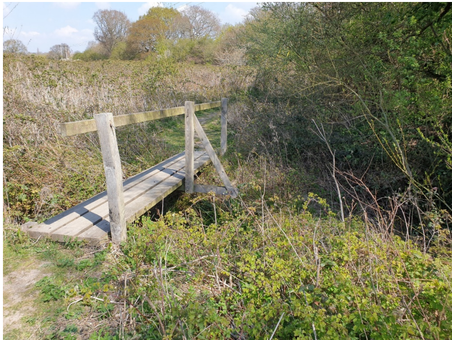
Plate 14: Pedestrian bridge from Area 4 into Area 1
