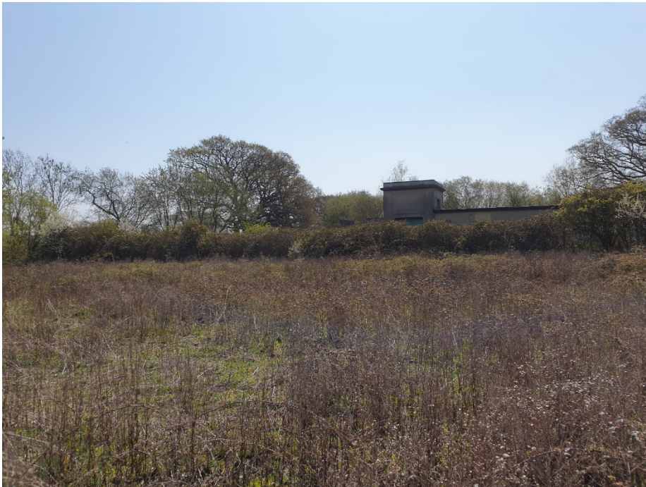
Plate 18: Within the south western part of Area 1 looking at electricity sub-station (on opposite side of railway line).
