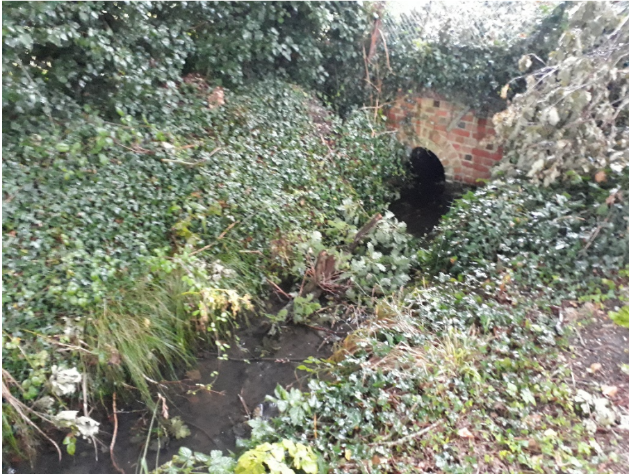
Plate 11: Ditch flowing beneath adjacent railway line.
