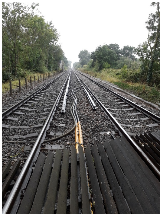
Plate 12: Photograph of the railway line along the southern boundary taken from the pedestrian level crossing.
