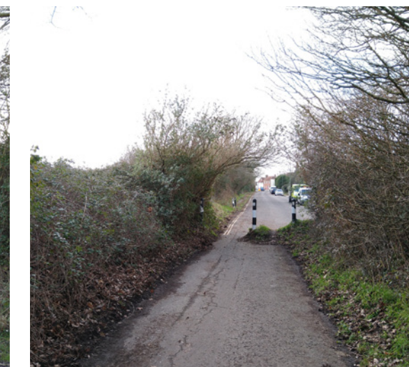
Existing cycle path along northern boundary (at connection with Old Arundel Road)
