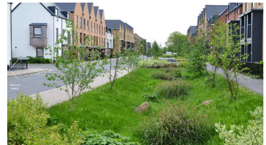
SUDS swale in residential areas
