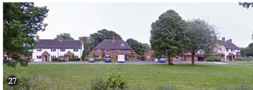
27 Semi-detached houses on east side of Brooks Lane, facing onto green space
