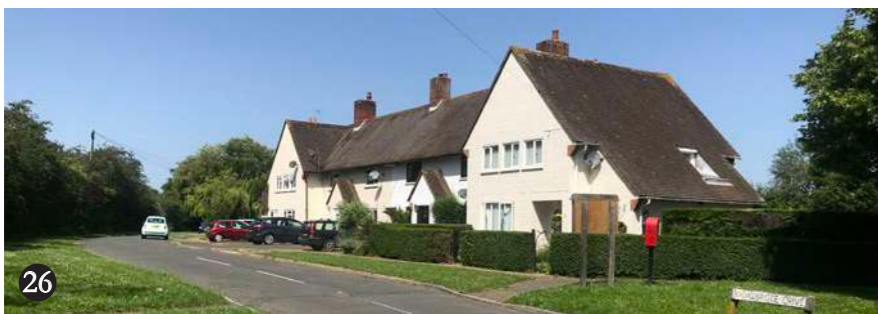
26 Terrace on Broadbridge Drive with distinctive gabled fronts and catslide roofs
