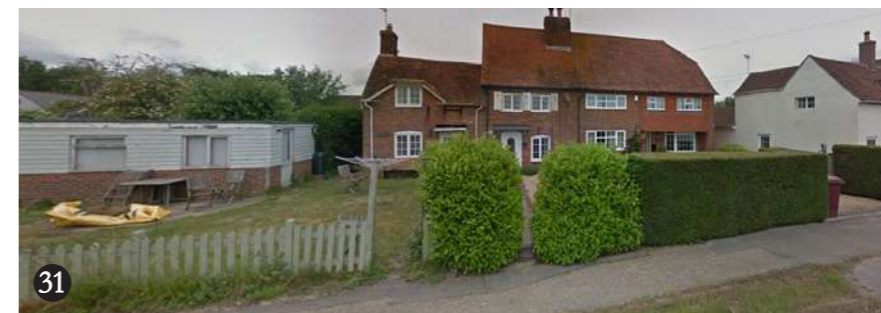
31 Properties off A259 Main Road, south of Ham Farm
