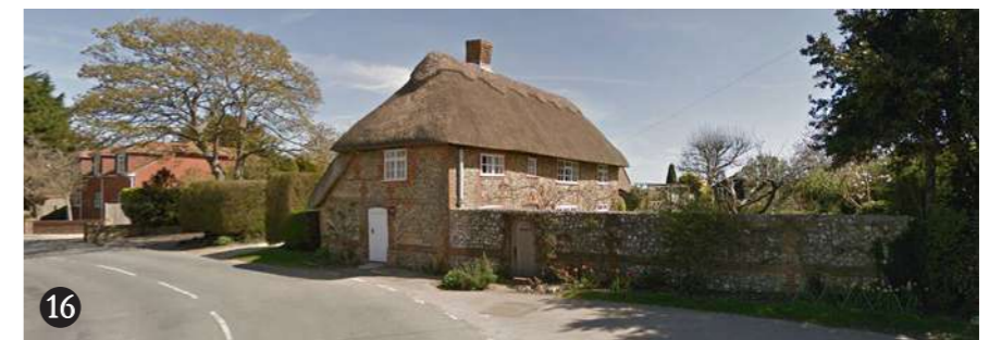
Grade II listed Laurel Cottage (listed as Laurel House) on Walton Lane, Bosham
