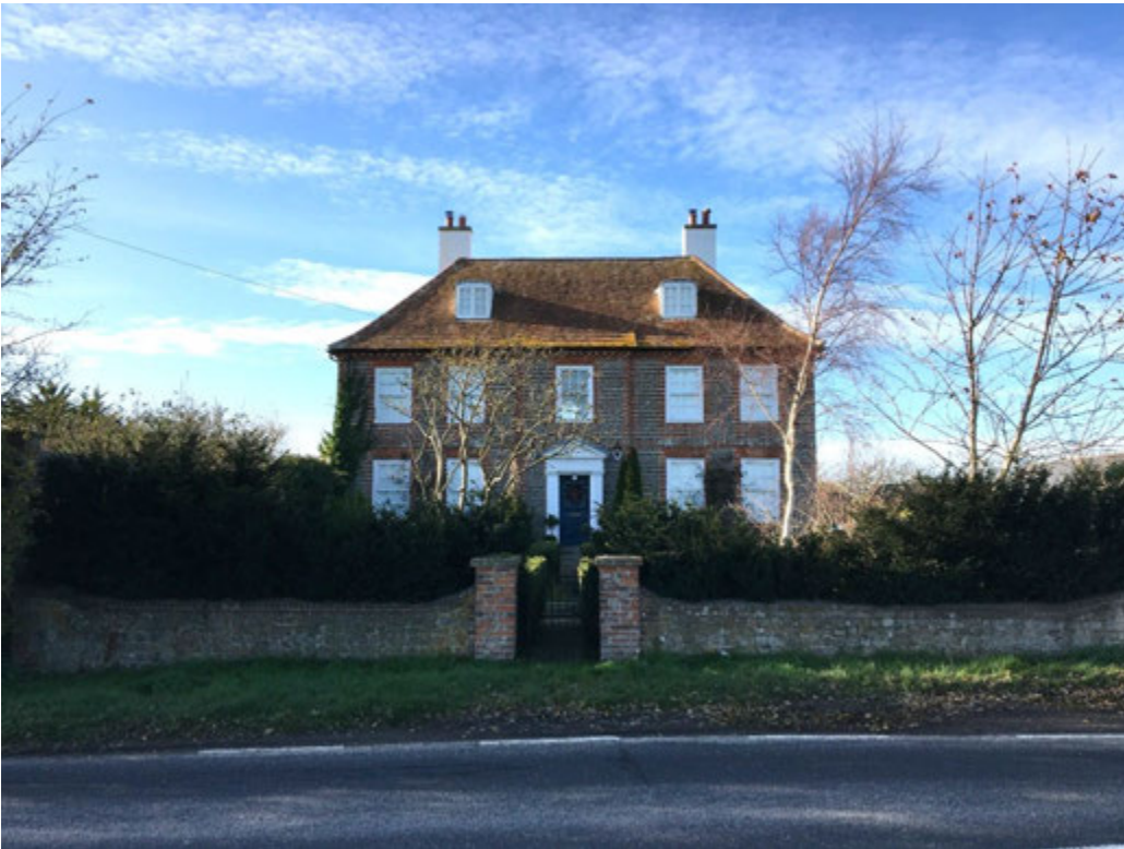
Figure 18: Coles Farmhouse, Grade II, viewed from Chichester Road.
